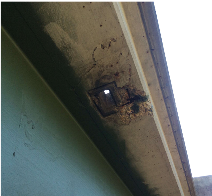
PHOTO 4 Description Spalls at drains
