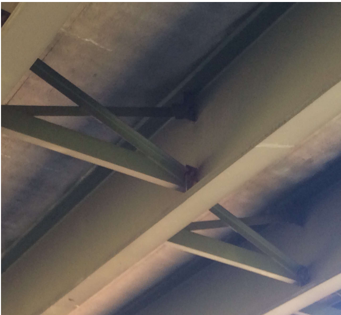
PHOTO 1 Description Missing bolt 3rd diaphragm span 4 bay 3
