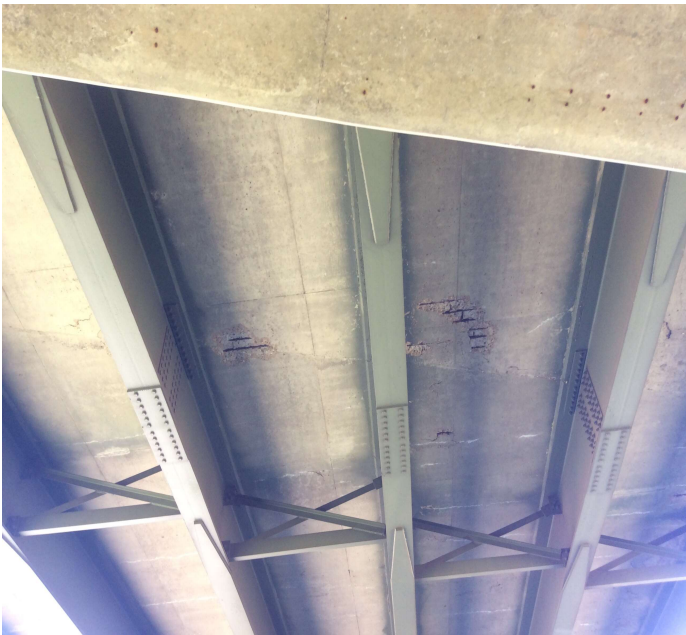
PHOTO 3 Description Span 2 all bays spalls with rebar
