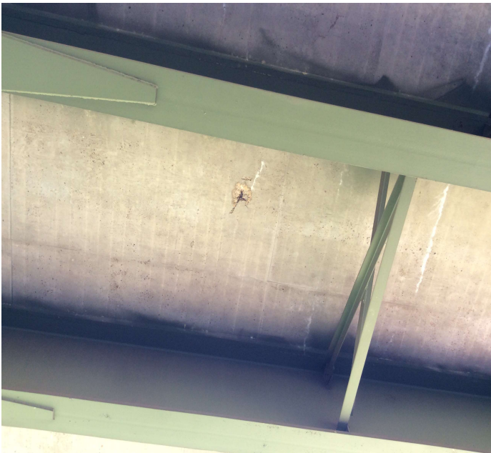
PHOTO 1 Description Span 3 spalls bottom of deck
