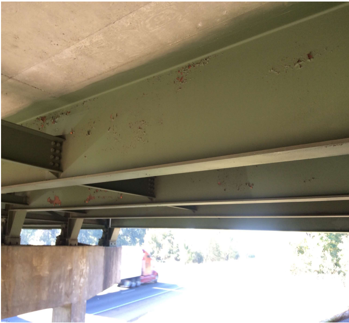
PHOTO 1 Description Paint peeling in various locations
