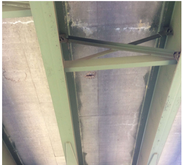
PHOTO 2 Description Span 3 bay 2 spall
