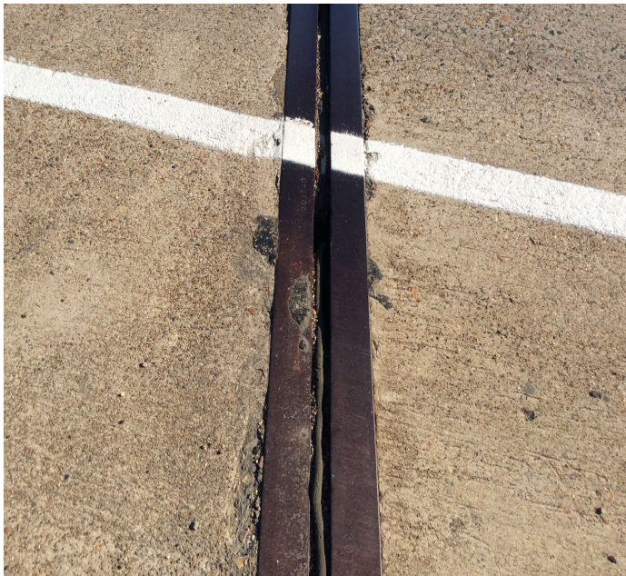
PHOTO 1 Description Bent 2 joint 1 foot missing at left white line
