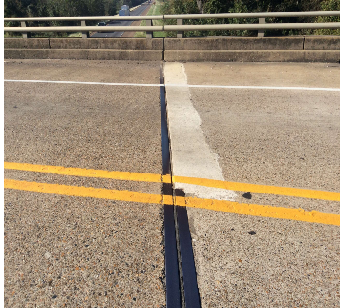
PHOTO 5 Description Bent 5 joint deterioration
