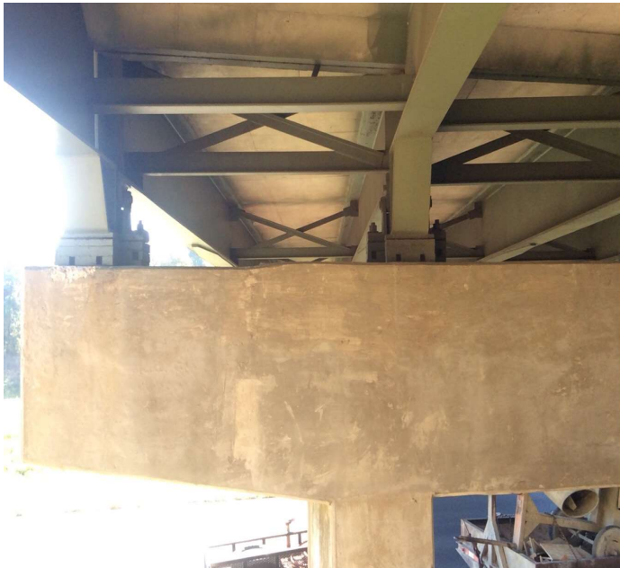
PHOTO 1 Description Bent 5 cap north face. Crack under beam 4, 5, and 6 and spall under bent 6 bearing
